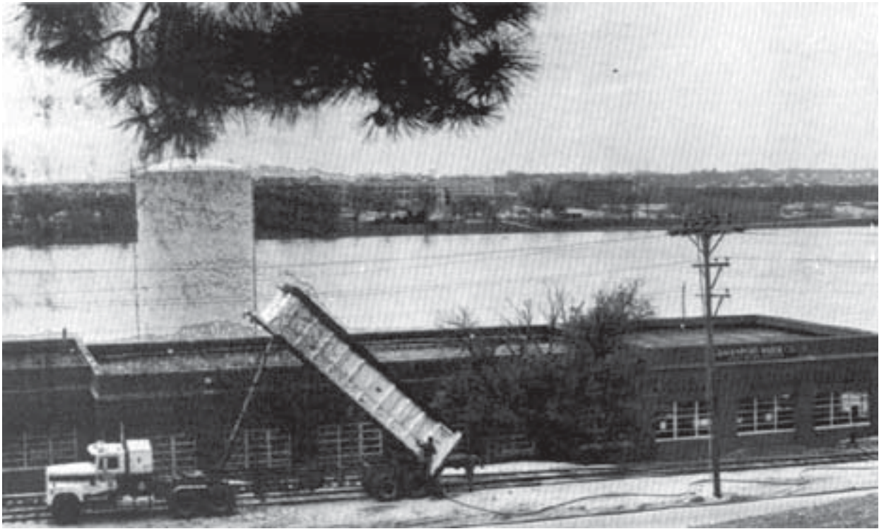
A 40,000 lb capacity dump truck delivers granular carbon to the Davenport Water Company plant on the Mississippi River. The facility supplies clean and safe drinking water to 126,000 consumers in Davenport, Riverdale and Bettendorf, Iowa.
